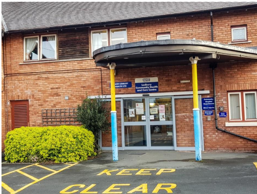
Figure 26 - Ledbury Community Health and Care Centre
